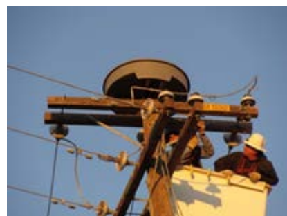
Installation of Osprey Nesting Platform
