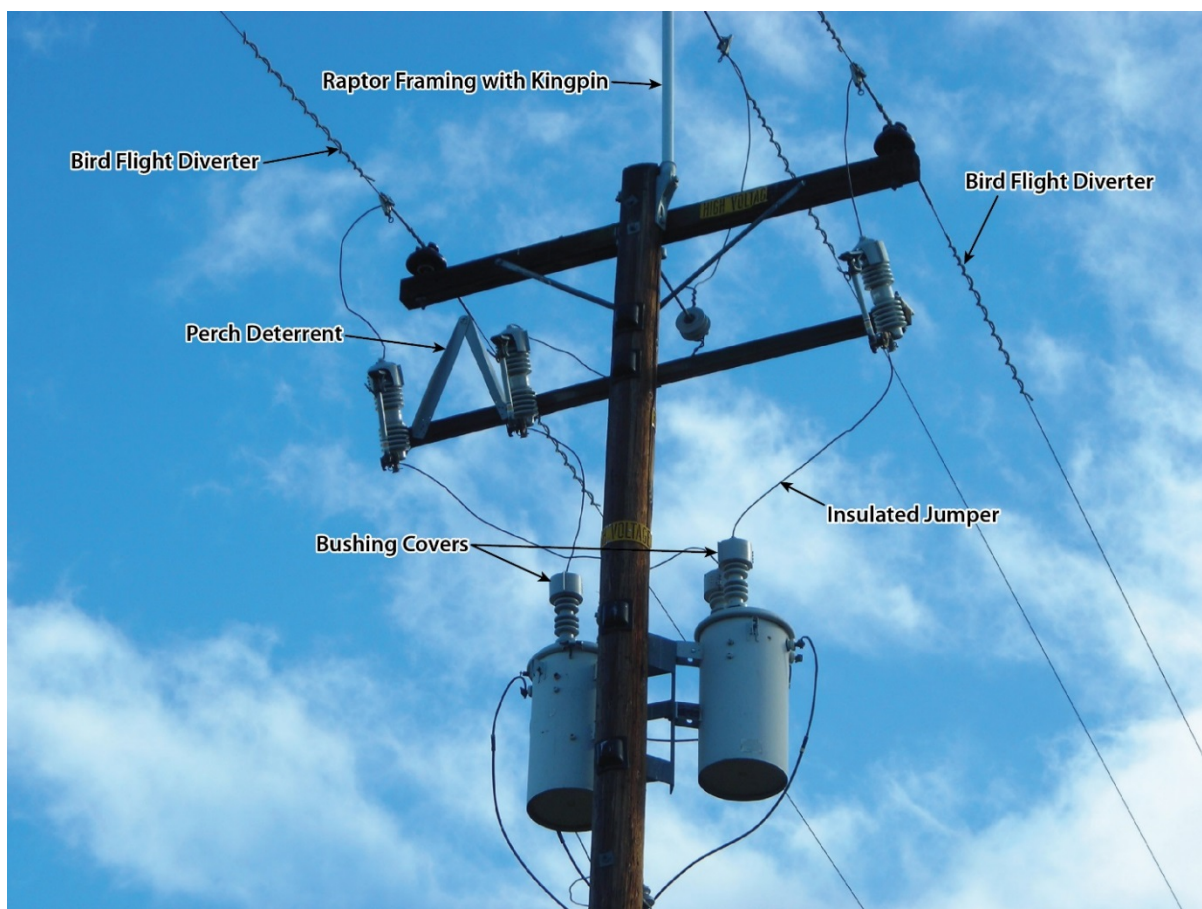
Figure 3. Important Avian Protection Hardware on Electric Facilities
